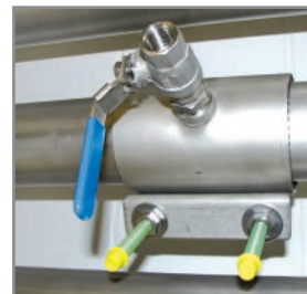
B Spot drilling collars
